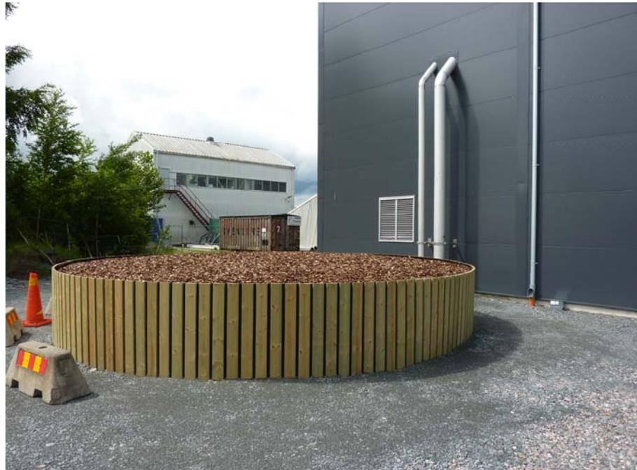
*Figure – Small bio filter for cleaning of carcinogenic trimethylamine from a plant for modified starch for the pulp and paper industry in Sweden. This filter is stage to accept various operation modes. It will accept flows from 400 – 2000 m<sup>3</sup>/h.*
