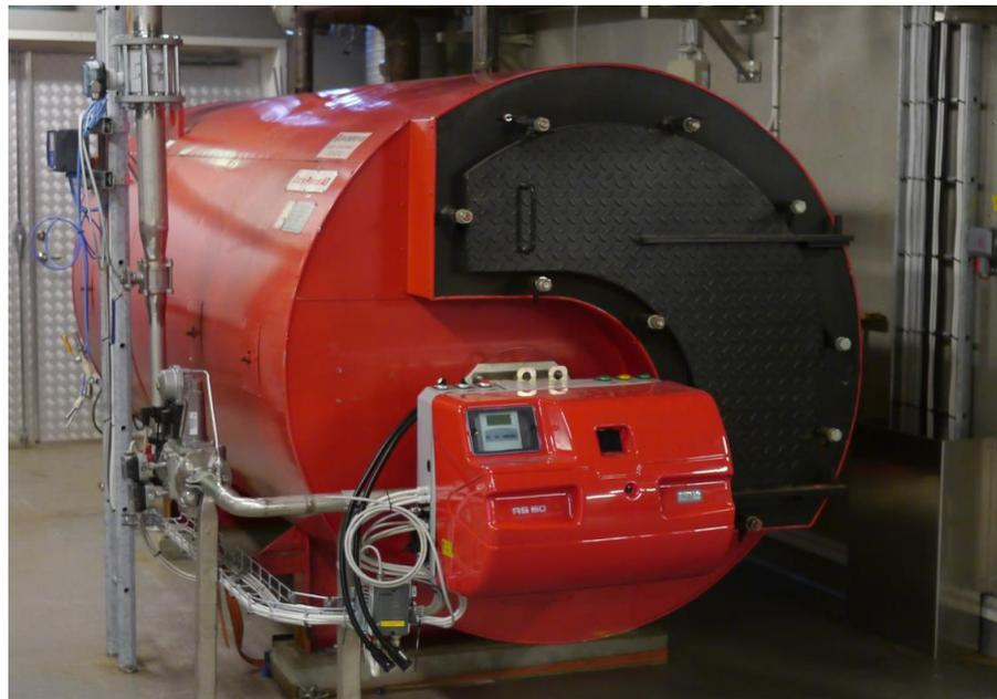
*Photo – Gas burner mounted on the hot water boiler*
