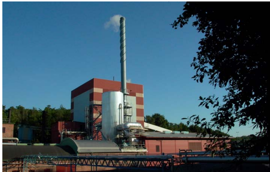
Figure – Perstorp AB. In the front a 330 m 3 silo for storage of animal waste and a wet electrostatic precipitator. In the background the boiler house for the 55 MW boiler.
