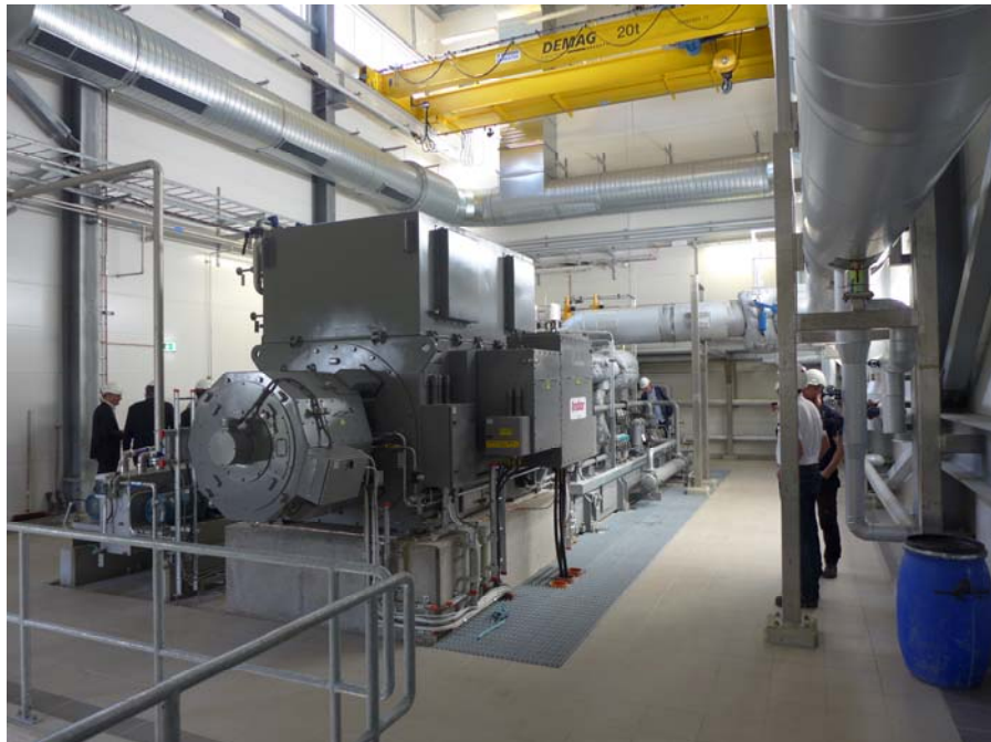
Figure – Turbogenerator installation in Nybro Waste to Energy plant.
