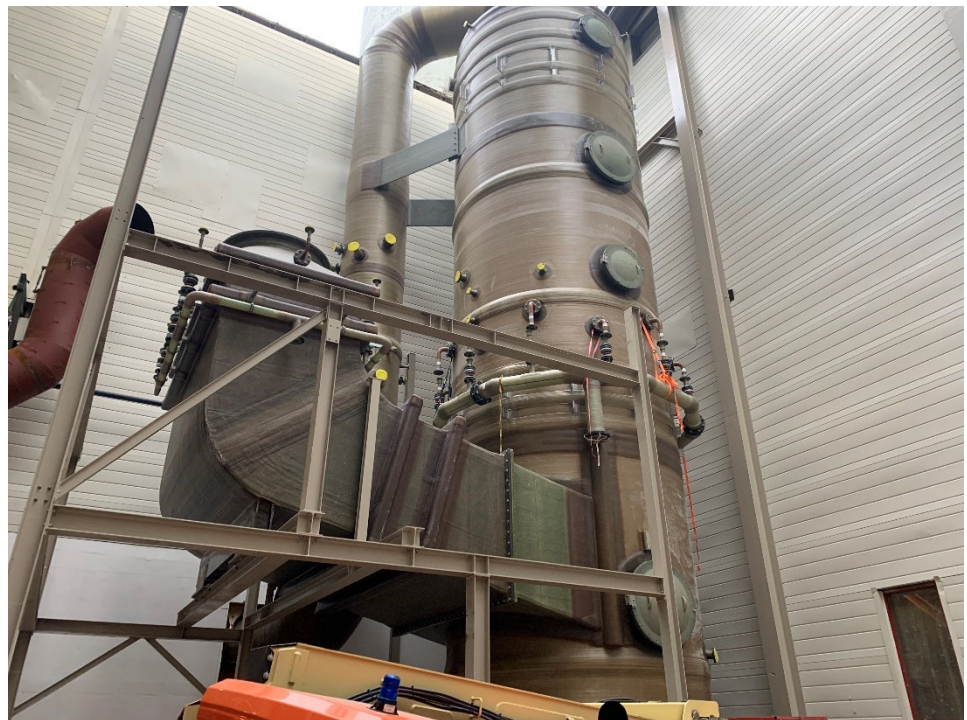
Figure – Scrubber tower installation, Lidköping.
