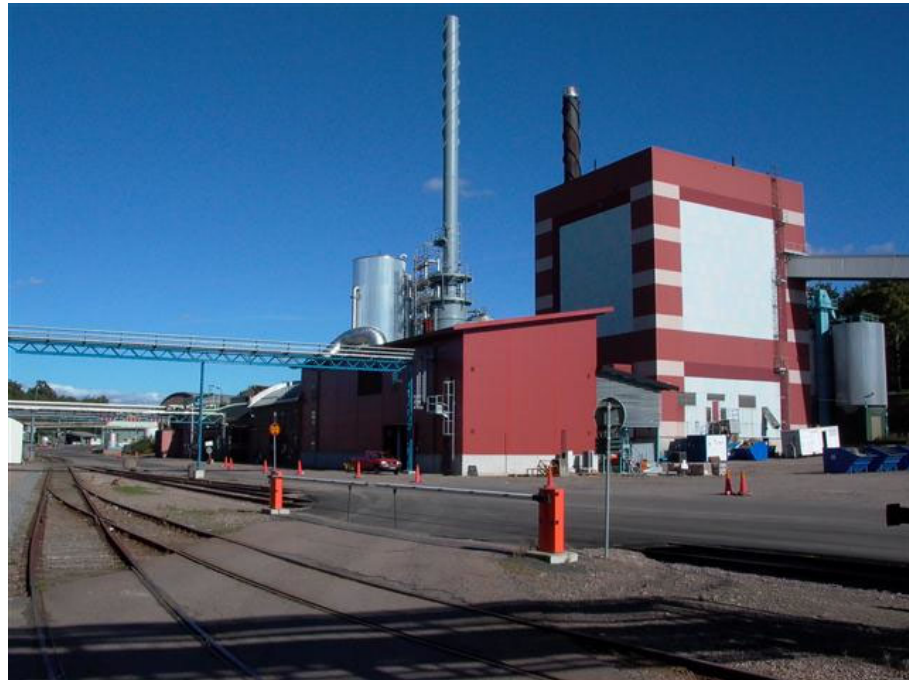
Perstorp, Sweden. Hazardous waste incinerator with WESP and animal by-products silo in the foreground. 55 MW CFBC in the background.
