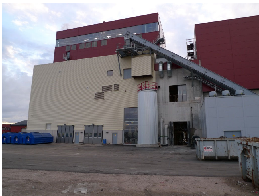
Bio-El Fredrikstad. CHP 20 MW th 6 MW el . Also, possible to operate with vacuum condenser.
